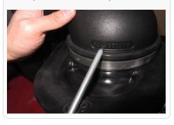
25. Once aligned tighten down the down clamp.
