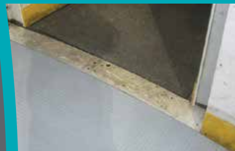
Panels Cut and Finished to Exactly Fit Dasher Boards
