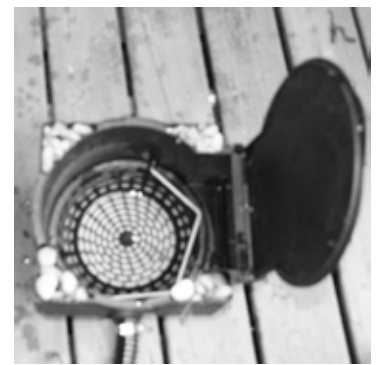
F) Add gravel in the corner pockets for weight.
