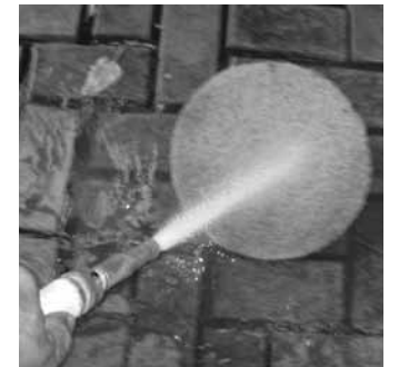
Skimmer Pad - The fiber mat should be inspected and rinsed off.
