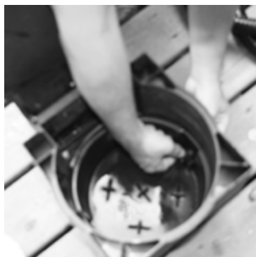
B) Secure with locknut.
