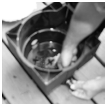
A) Insert barb adapter to the "pump side" of skimmer.
