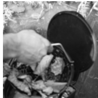
Basket - Debris and leaves collect inside the skimmer in a basket. Open lid, remove and clean basket.
