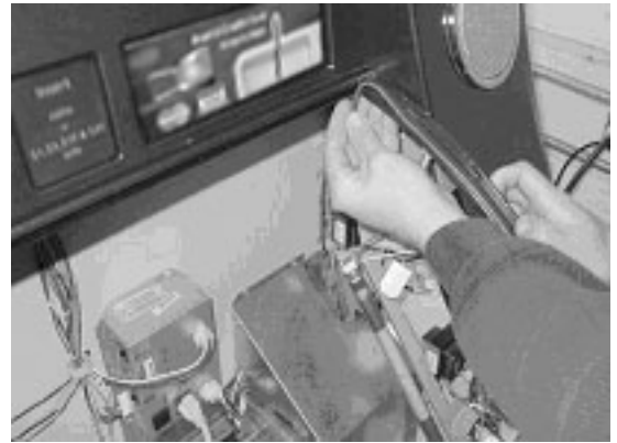
Figure 15 - Wrap Tape Over Flange Top
