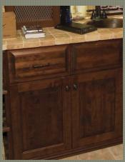
9) Cabinets and Drawers: You can choose a variety of door options: raised panel, radius raised panel, flat panel, glass, or mesh inserts. The material behind the doors can be made of either solid edge-glued wood or veneer plywood. WCI uses high quality, 110 degree, concealed European hinges on all of our doors. The drawers have ball bearing, full extension slides with 1" overtravel.
